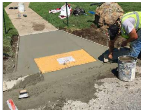
Figure 3: ADA Ramp Construction in Broken Arrow
