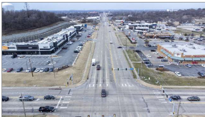
Figure 3: Kenosha Street at Lynn Lane Looking West
