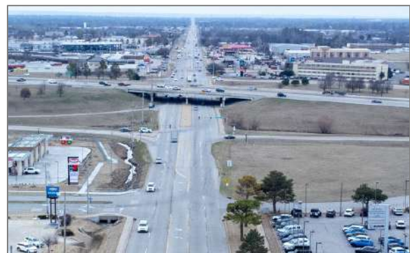
Figure 11: Broken Arrow Expressway
