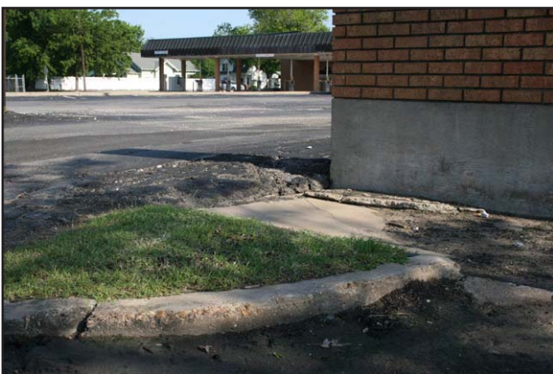
055 - North alleyway and sidewalk on W El Paso St
