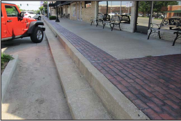
105 - East side step curb and brick pavement on 100 Block of N Main St
