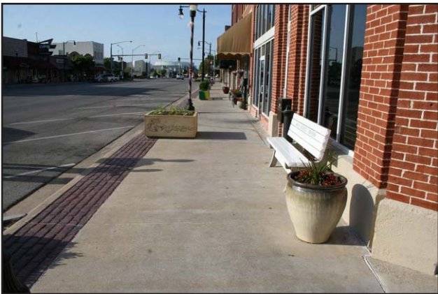
035 - West side sidewalk on S Main St at 200 S Main St
