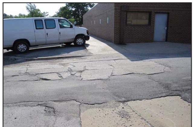
088 - South side alleyway and sidewalk on E Commercial St
