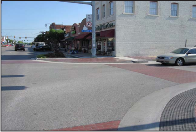
081 - Northeast corner of S Main St & E Dallas St
