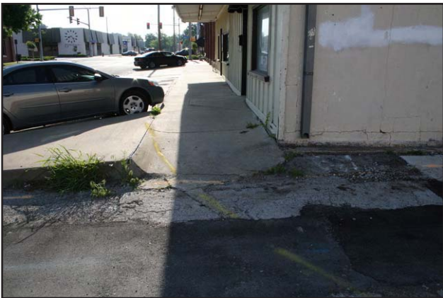
029 - South side alleyway and sidewalk on W Commercial St
