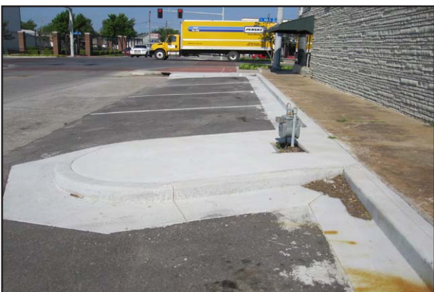
103 - North side parking curb and sidewalk on E Broadway Ave
