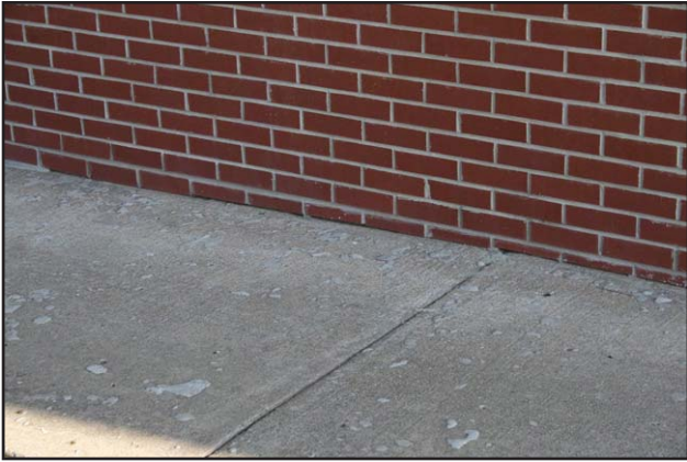
017 - North side sidewalk and building facade on W Commercial St
