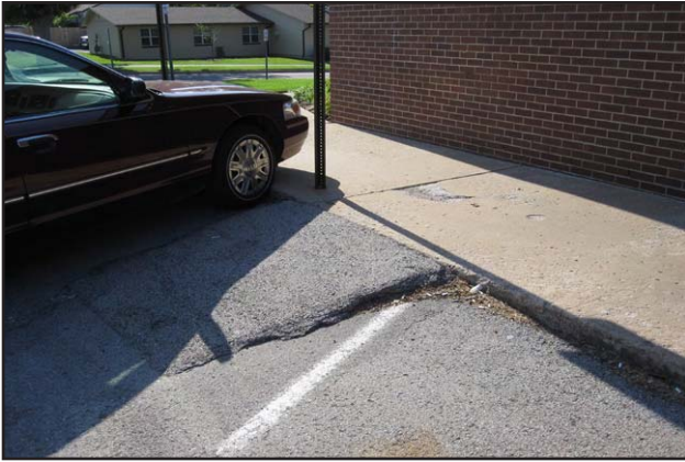
089 - South side curb ramp and sidewalk on E Commercial St
