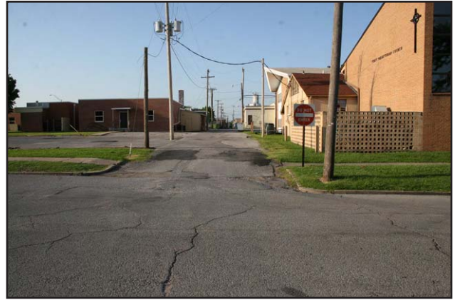
002 - South side alleyway on W College St
