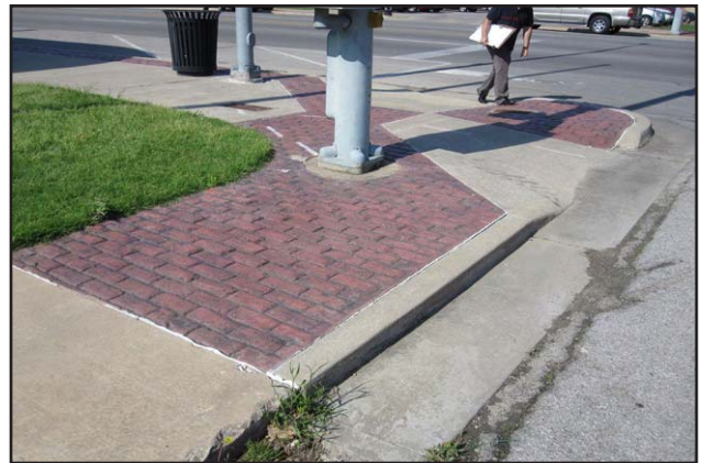
108 - Southeast corner of N Main St & E College St
