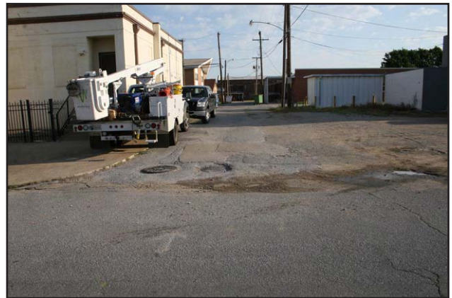
006 - North side alleyway on W Broadway Ave
