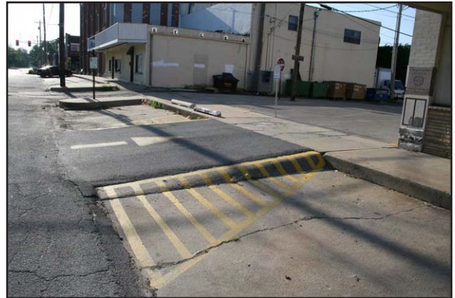
028 - South side driveway, sidewalk, and alleyway on W Commercial St
