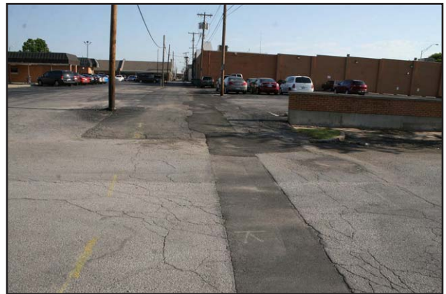
054 - North alleyway on W El Paso St
