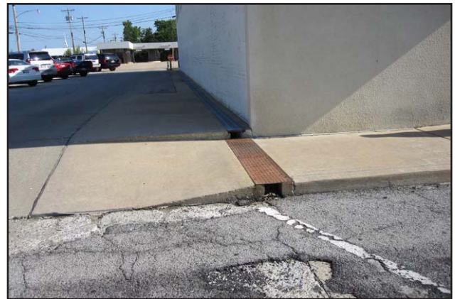
094 - North side driveway and sidewalk on E Commercial St
