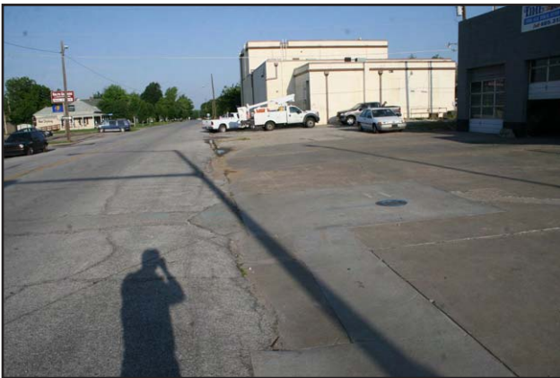
005 - North side driveway and sidewalk on W Broadway Ave
