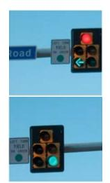
This protective/permissive left-turn signal provides the motorists with a period of time where left-turns with an arrow can be made without encountering conflicting traffic, after which, motorists are presented with a green ball where left-turns can be executed between gaps of through traffic. This type of left-turn can be used when:
