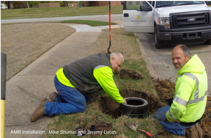
AMR Installation: Mike Shumar and Jeremy Lucas
