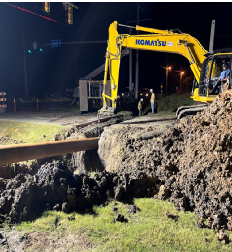
On the left: Repair & Construction crew working overnight to install water line at Garnett Rd
