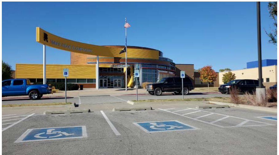
The new elementary school is located in an isolated area and only accessible by cars and school buses
