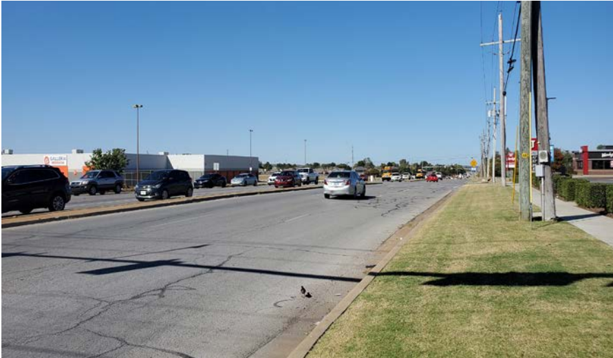
Existing 6-lane, arterial County Line Road (looking north)
