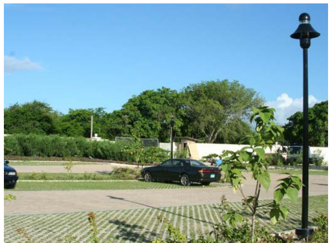
Grasscrete parking to help reduce impervious surface
