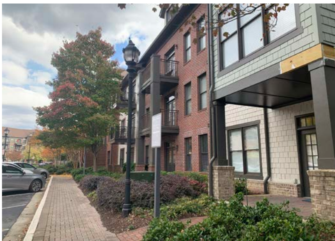
Multi-family building with a deeper setback to accommodate building articulation and landscaping
