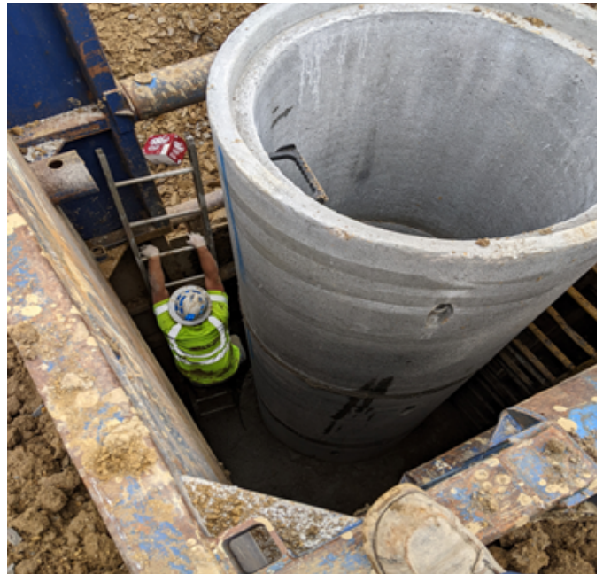
Dakota Orcutt checks the grouting of a manhole at 37th Street.
