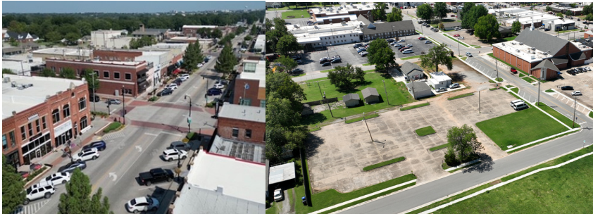
The Rose District parking lot project has been awarded. KJRH reported on the development noting the inclusion of pavement, fencing, landscaping, irrigation, signage and light poles in the improvements.
