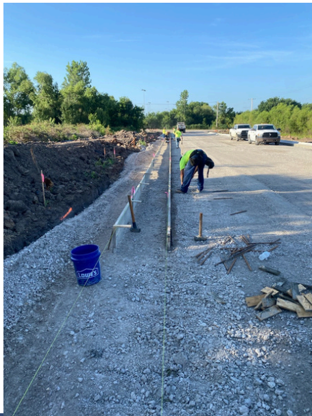
The construction of 43rd Street on the east side of Rosewood Elementary School near Events Park is progressing. Streets crews have cleared the land to the railroad and poured 400 feet of new curb with another 400 feet ready to pour.
