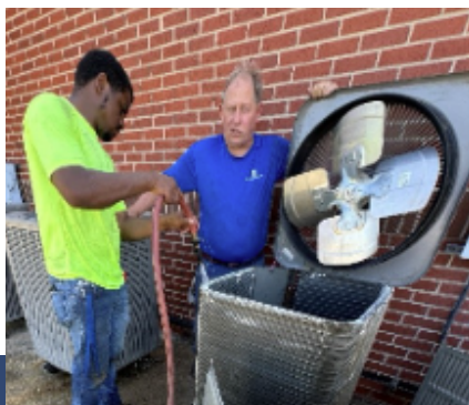
Don and Andrew cleaning condenser units at Fire Station 5.
