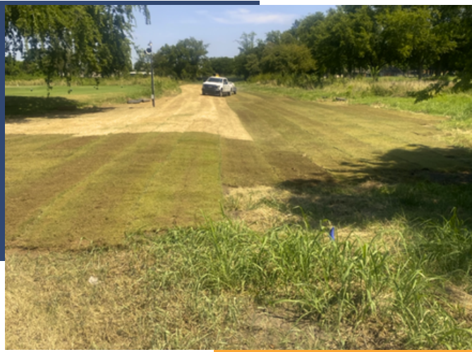
(Upper left) - Drainage improvements at Battle Creek Golf Course
