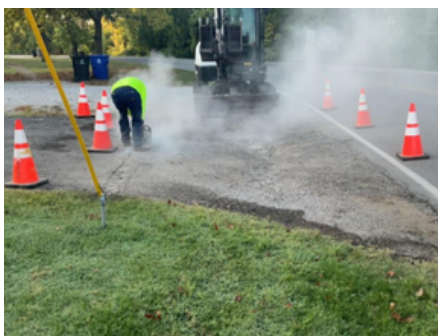
Stormwater/Storm Drain work completed on 1st Street with new concrete.
