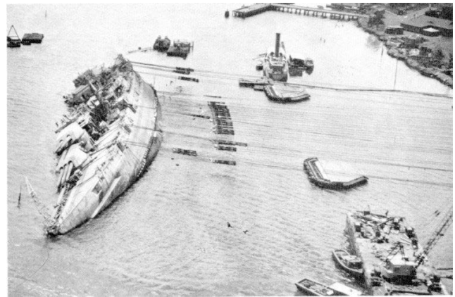
Righting Oklahoma – The complex task was contracted to the Pacific Bridge Company under Navy supervision.
